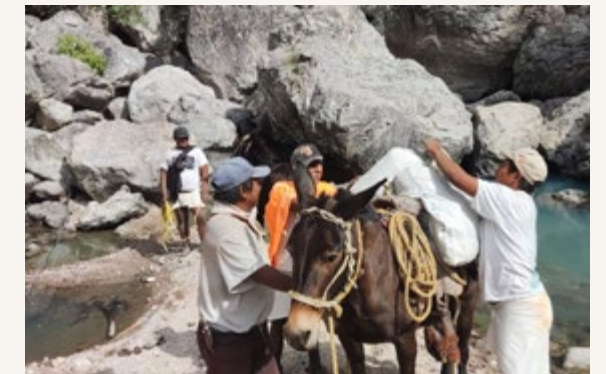
Community members transport materials for the construction of water storage tanks
